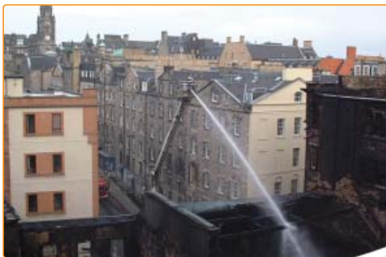
The Cowgate fire spread quickly due to hidden chimney flues and ceiling voids.
