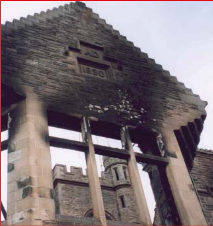
Hartwood Hospital in Shotts, Ayrshire, following severe damage by fire. © Crown copyright.
