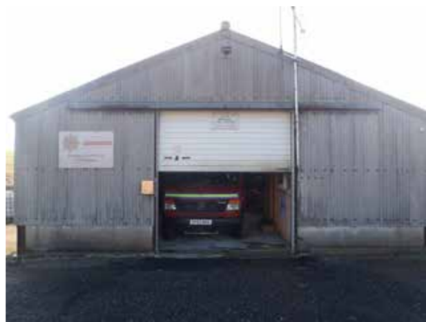
Bressay Community Fire Station
