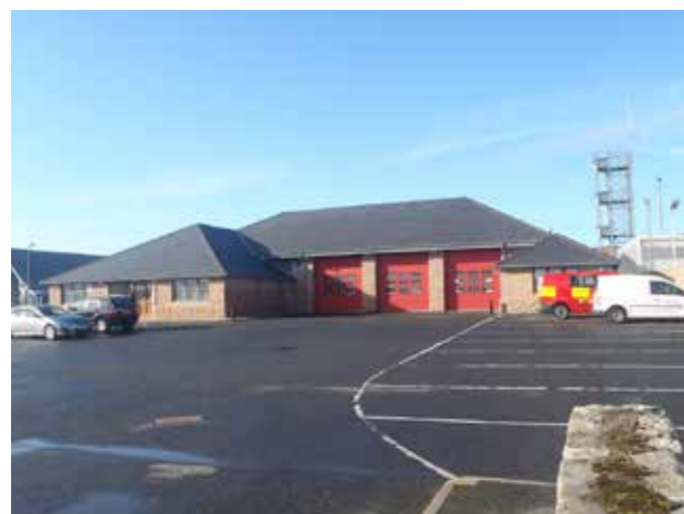
Lerwick Community Fire Station
