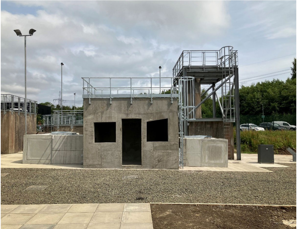
Image 5 – Structural collapse simulator facility investment
