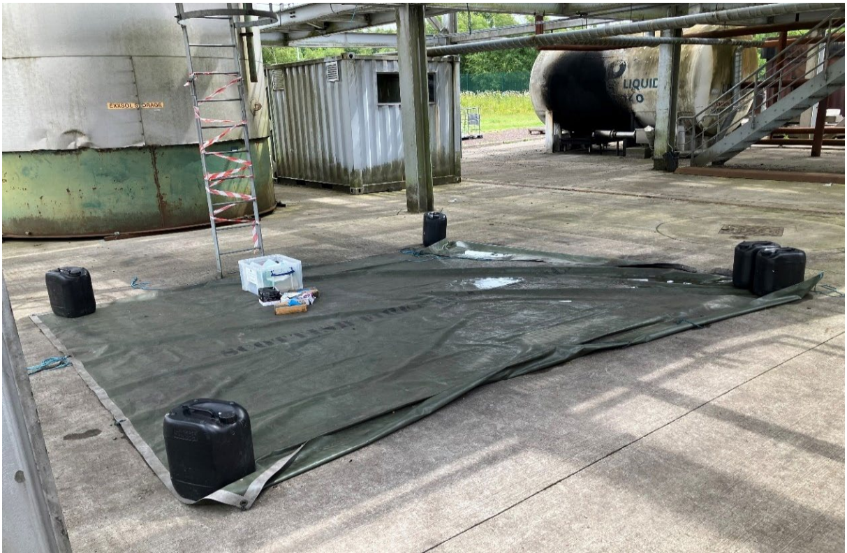
Image 6 – Typical example of temporary Contamination Control measures.
